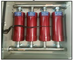
Water gets conditioned if the Flow rate does not increase more than 600 Liters per Hour. Hence our R&D team have developed a Multi-Flow Design concept where Flow of water above 600 Liters per hour splits to multiple candles (While each candle processes 600 Liters per hour) in order to ensure Hard Water gets conditioned to Soft Water.
